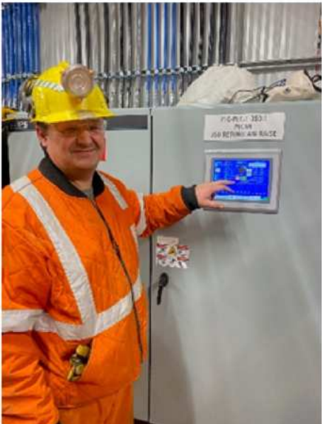
Powering up the new 350 Return Air Raise for the first time!
